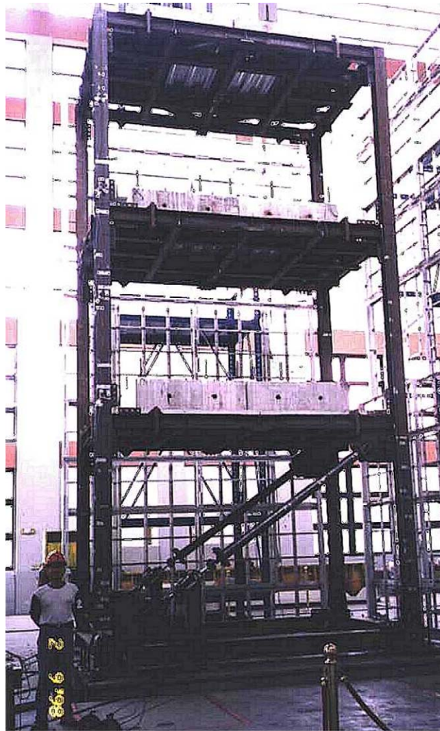
Fig. 8. Three-story full-scale building on the shake table of NCEE.
